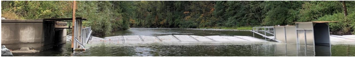
Figure 8: Two-passage counting fence configuration with wide passageways located mid-river and at the bulkhead, first piloted in 2019.
