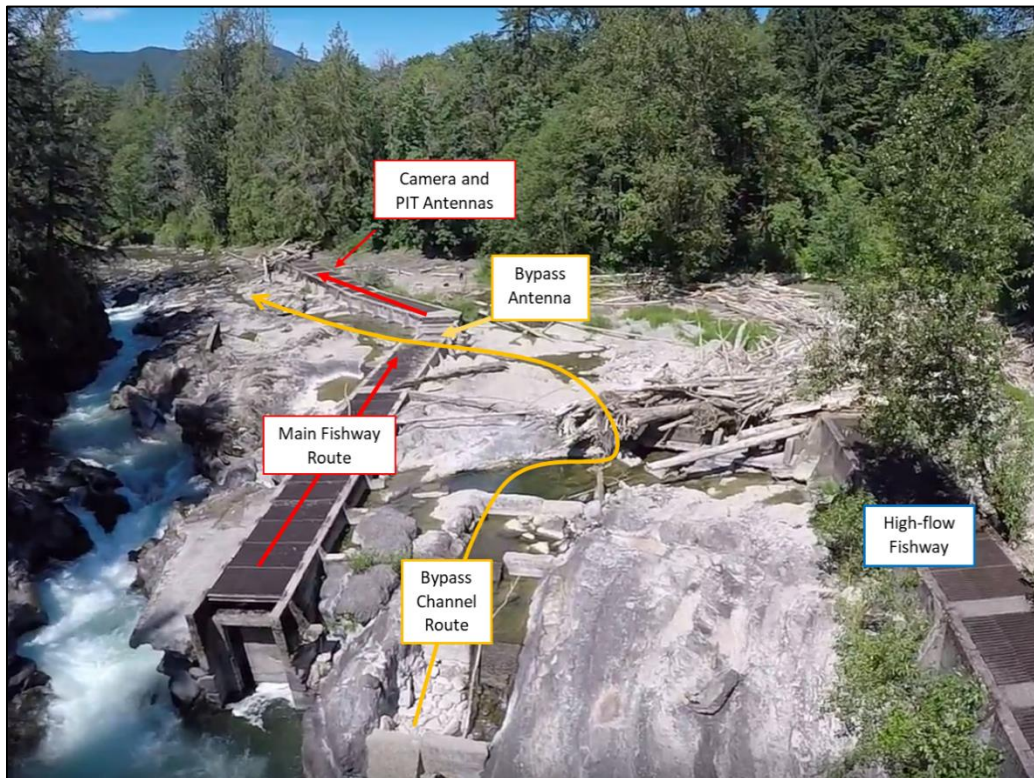
Figure 11: Skutz Fishways, bypass channel, migration routes, and monitoring equipment.
